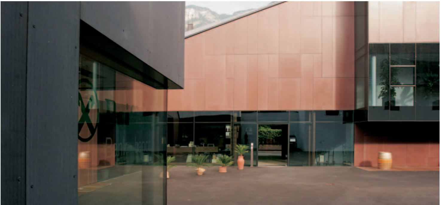
GLASS FIBRE REINFORCED CONCRETE FACADE © Darren Penrose
